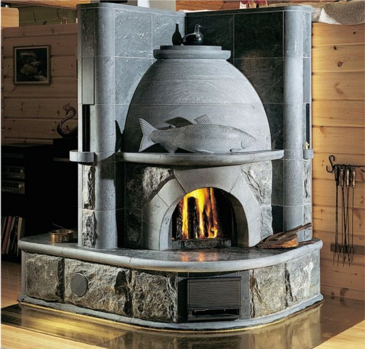
FIGURE 2.11. Here is a modern version of Kate Seredy’s “beehive.” This custom soapstone heater in Finland sports a heated bench and a carved fish on the mantel. The “beehive” shape contains the firebox and a secondary chamber above a throat. The exhaust travels from the upper part of the dome down into the heated benches and then up into the tall rectangular elements in back before exiting into the chimney flue at center left. Photo courtesy of Tulikivi Corporation.
