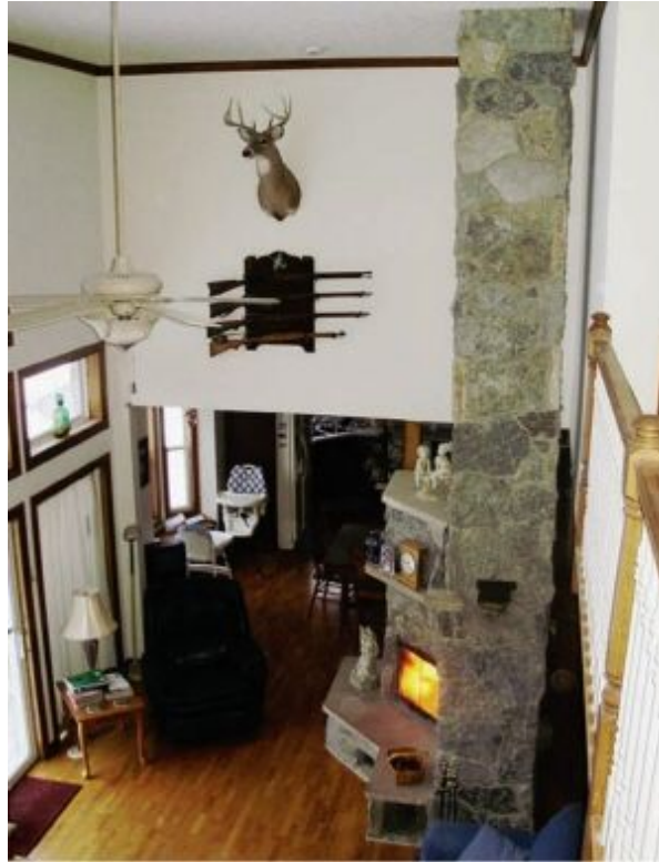
FIGURE 5.3. A masonry heater is best placed centrally in the main living area of the home. This bluestone heater serves as a room divider between the eat-in kitchen, the living room, and a hall leading to other parts of the house. The view is from the balcony and shows the entire 18-foot-tall chimney. The heater itself is six-sided with the chimney coming off one of the triangular sides. Another view of this heater is in the photo at the beginning of part 4.
