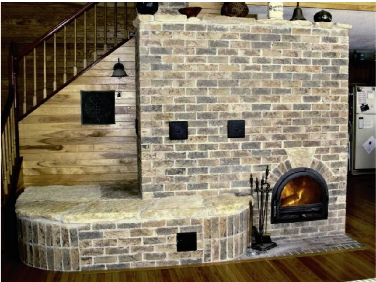
FIGURE 3.5. This brick-faced masonry heater has a massive heated sitting area to the left. The exhaust travels through flues inside the bench directly after leaving the firebox. The curved shape of the bench expands the walkway from the stairs on the left. Figures 4.6 and 5.1 show other views of this heater.
