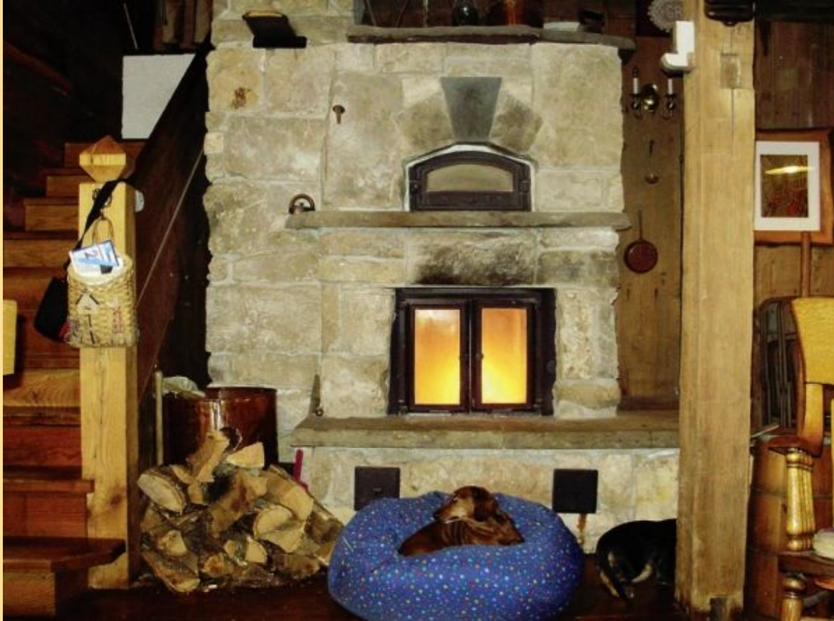
FIGURE 10.13. Lindsay Graham and his son Zach veneered this heater with local limestone and sandstone. It's now the primary heat source for the Graham household. This heater is also pictured in figure 6.35.
