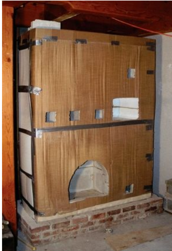
FIGURE 8.2. The inner life of this modular heater is wrapped, per manufacturer’s instructions, with cardboard. Veneer material is thereby separated from the inner life by a 1.4-inch gap. When the unit is used, the cardboard will disintegrate, leaving a 1.4-inch air gap. Photo by Wendell Short.
