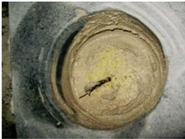
FIGURE 8.16. A view of the same cleanout seen in figure 8.15, this time through the soapstone opening as you would see it after the heater is done (minus the eventual soot door).
