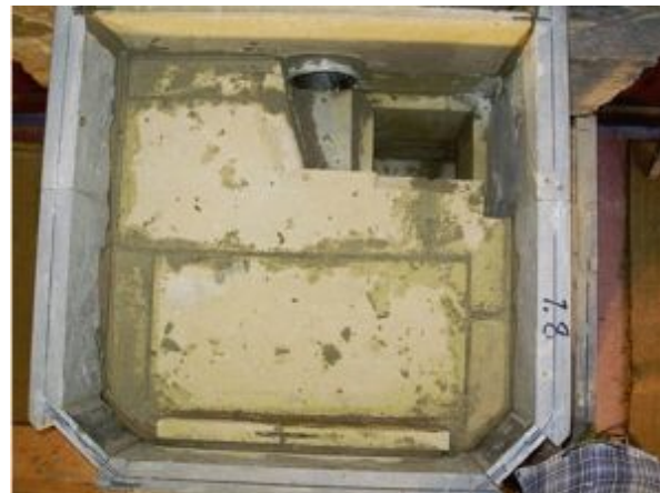
FIGURE 8.39. Note pins holding soapstone to soapstone, insulation board to soapstone, and a (difficult-to-see) mitered corner—all precautions to keep the inner life and the container operating together like one living being.
