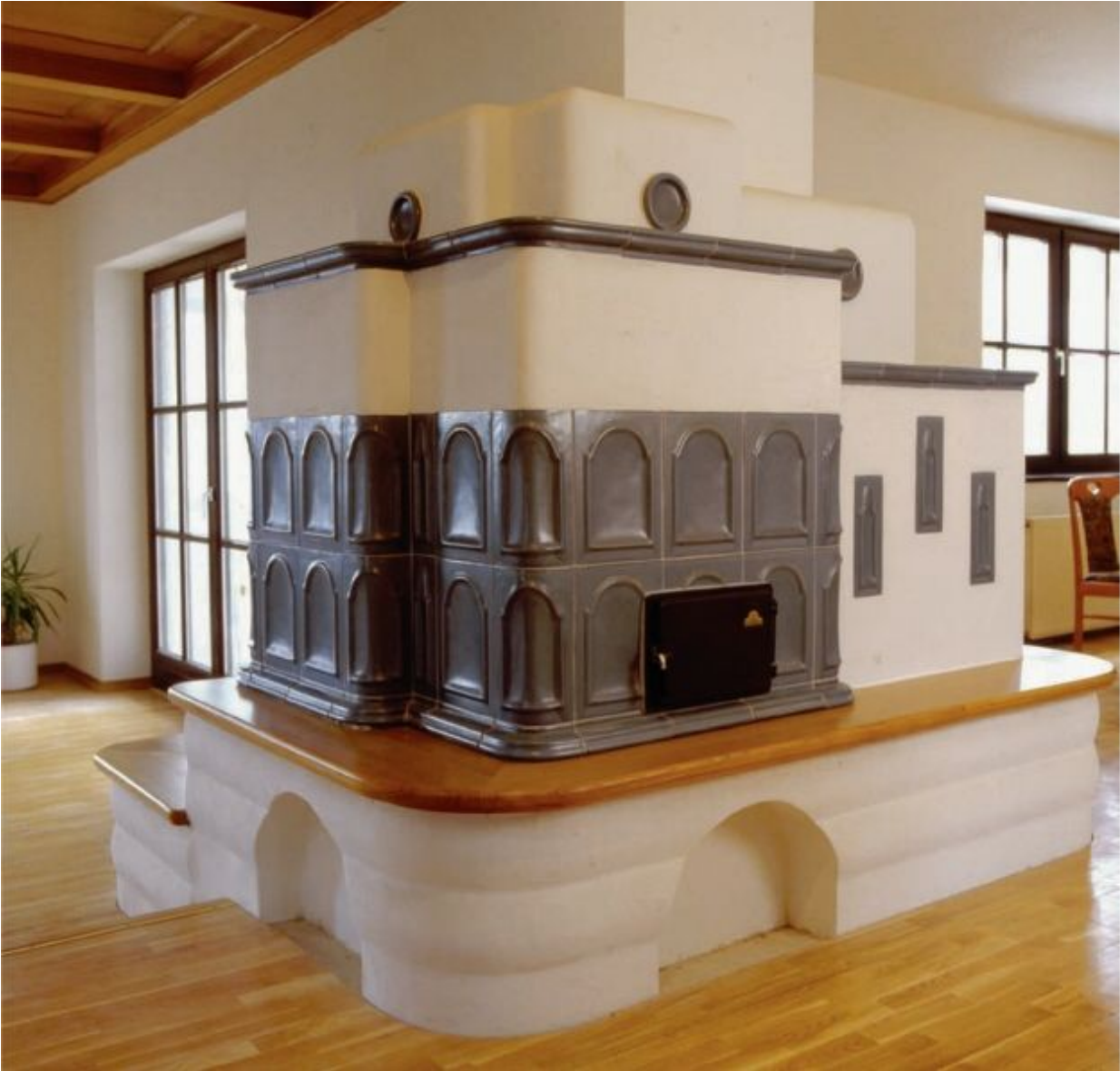
FIGURE 3.4. This stucco-and-tile masonry heater incorporates wood for the bench surfaces. Corners are gently rounded, giving the otherwise rectilinear elements a soft appearance. The black loading door gives the classic European look and hints at a small firebox. The shape of the tiles is a traditional one as well. Notice how the heater's bench steps down to the left to follow the level change in the room. Photo courtesy of Biofire, Inc.
