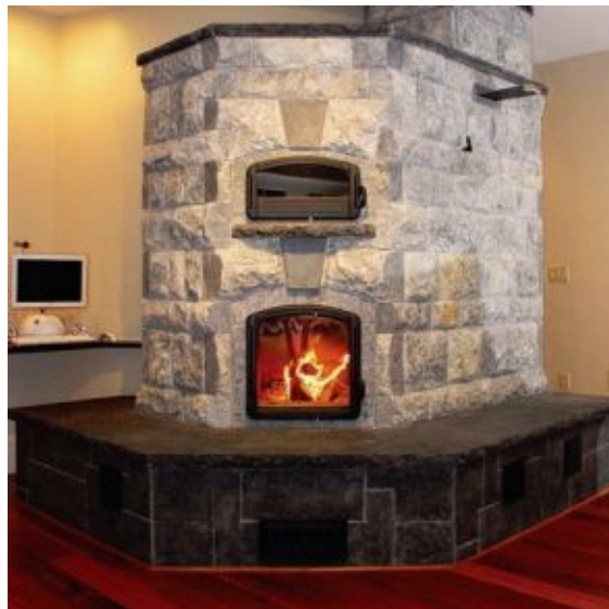
FIGURE 6.34. Here is a wonderful example of a finely crafted stone masonry heater. The dark granite heated benches and heater cap contrast with the lighter stone used on the main body of the heater. Photo courtesy of Maine Wood Heat Company.
