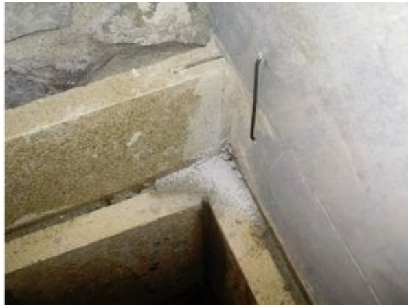
FIGURE 8.39. Note pins holding soapstone to soapstone, insulation board to soapstone, and a (difficult-to-see) mitered corner—all precautions to keep the inner life and the container operating together like one living being.
