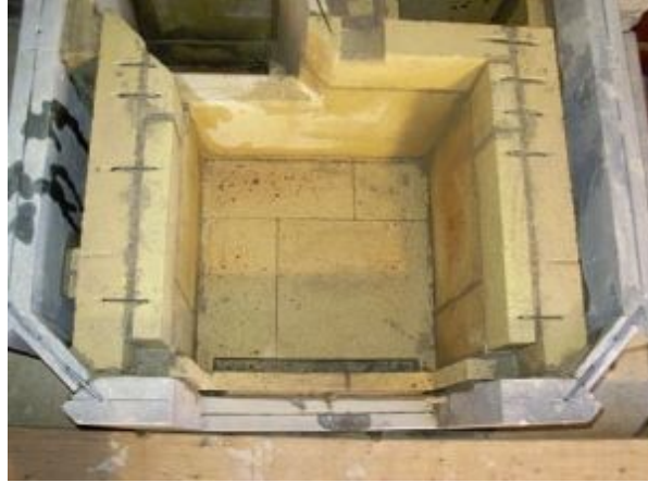
FIGURE 8.32. The completed firebox. Visible just inside the door opening is the air-intake slot that later will have a cover/ deflector built over it to keep out ash and coals. In the middle back of the picture is the little gas slot—a direct connection to the flue to guarantee no collection of flammable gases. The outburn is complete, and the door opening is being lined with refractory to protect the soapstone from direct heat from flames. Note that all inner and outer firebox slabs are pinned together to create a fully integrated assembly that will stay together under expansion and contraction.
