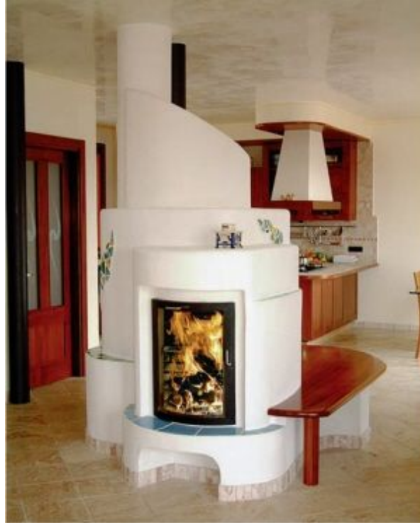
FIGURE 5.11. This finely sculpted stucco heater has no walls around it to hinder its heating ability. A simple but curved wooden bench follows the contours of the heater, and delicate tile accents add just a little color. Every curved surface here will radiate heat like the sun. Photo courtesy of Biofire, Inc.
