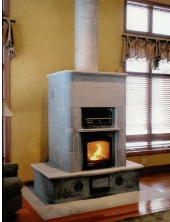
FIGURE 6.38. Soapstone almost always has a gray appearance on masonry heaters, but it often has marble-like graining that gives it great character and enduring beauty. The wing benches here are not heated. Notice cylindrical stones encasing the chimney. This would be difficult to do with most other stones. Tulikivi stove by Masonry Heater Store.
