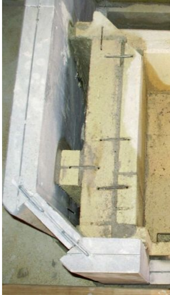
FIGURE 8.27. A large air gap between the container of soapstone and the firebox walls (or flue walls) permits convective in addition to radiant heating of the exterior. A small air gap of 1.4 to 1.2 inch would, instead, serve as insulation against heat transfer.
