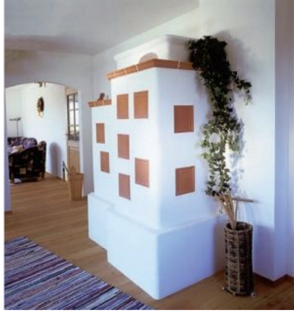
FIGURE 1.6. Tile trim decorates this stucco heater in the center of a home. Notice there is no visible fire or loading door facing the room. In Europe in the old days, heaters like this were sometimes fired by servants through a fuel-loading door in a back hallway or the kitchen. With a heater like this, the attraction is in the design and color as well as the gentle heat, rather than the fire itself. Photo courtesy of Biofire, Inc.
