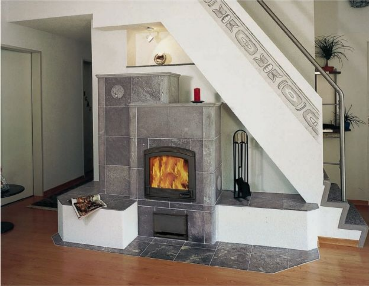
FIGURE 4.1. A small soapstone heater is tucked into a hard-to-use space. Sometimes a home's structural features introduce spaces that aren't very functional. This placement of a masonry heater shows how such an area can become a cozy, warm nook. The sitting areas of this one are not heated internally. The chimney flue is hidden in the wall behind the taller element of the stove. Photo courtesy of Tulikivi Corporation.
