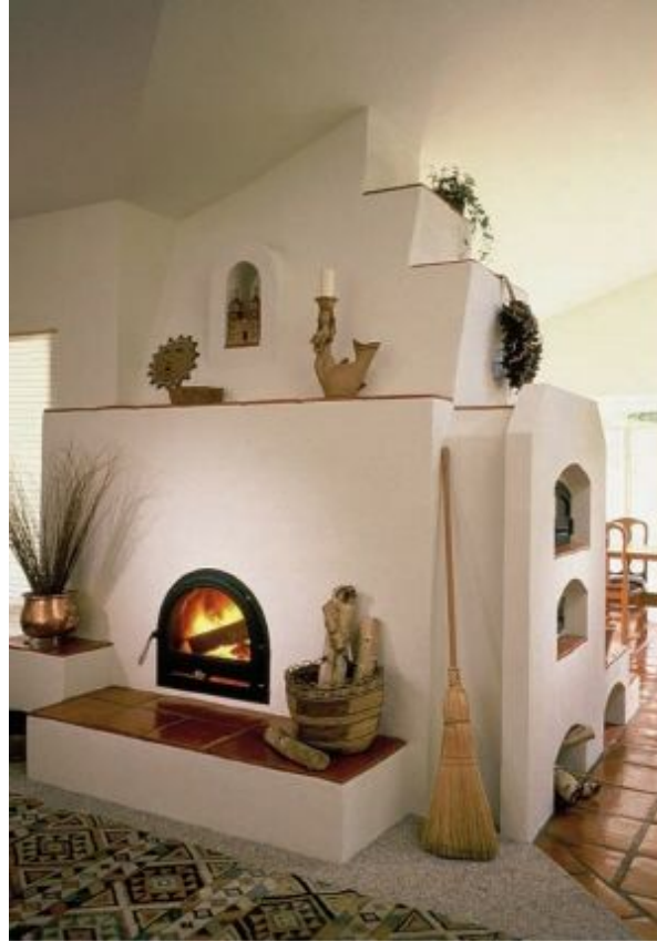
FIGURE 4.9. The front or firebox side of this heater has a lot of the traditional fireplace look, but you can also see the bakeoven door to the right, revealing that this is, indeed, something different. Figure 4.10 shows the other side of this masonry heater. Photo courtesy of Envirotech Masonry Heaters.
