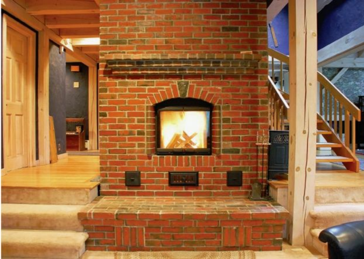
FIGURE 6.2. A brick, Finnish-style masonry heater often has the standard fireplace look that many homeowners desire. Notice the deep brick raised hearth and the ornate brickwork and arch around a square door, giving the appearance of a larger opening. Photo courtesy of Maine Wood Heat Company.
