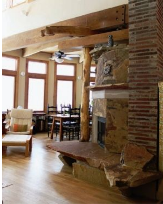
FIGURE 6.31. The chimney (far right) of this sandstone heater was built using long, thin Roman brick. Project by Maren Cooke and Ken Matesz; photo by Maren Cooke.
