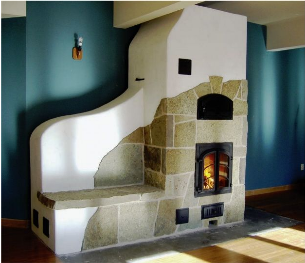
FIGURE 1.1. A masonry heater is a piece of functional art. Here stone and stucco are combined on the facade, and there is a heated sitting area. Notice how the left side of the tall element is sculpted to artfully miss the structural ceiling beam. The little black squares are ash cleanout doors and give a clue as to where exhaust and heat travel in a masonry heater. Designed and built by Stovemaster; photo courtesy of Alex Chernov.
