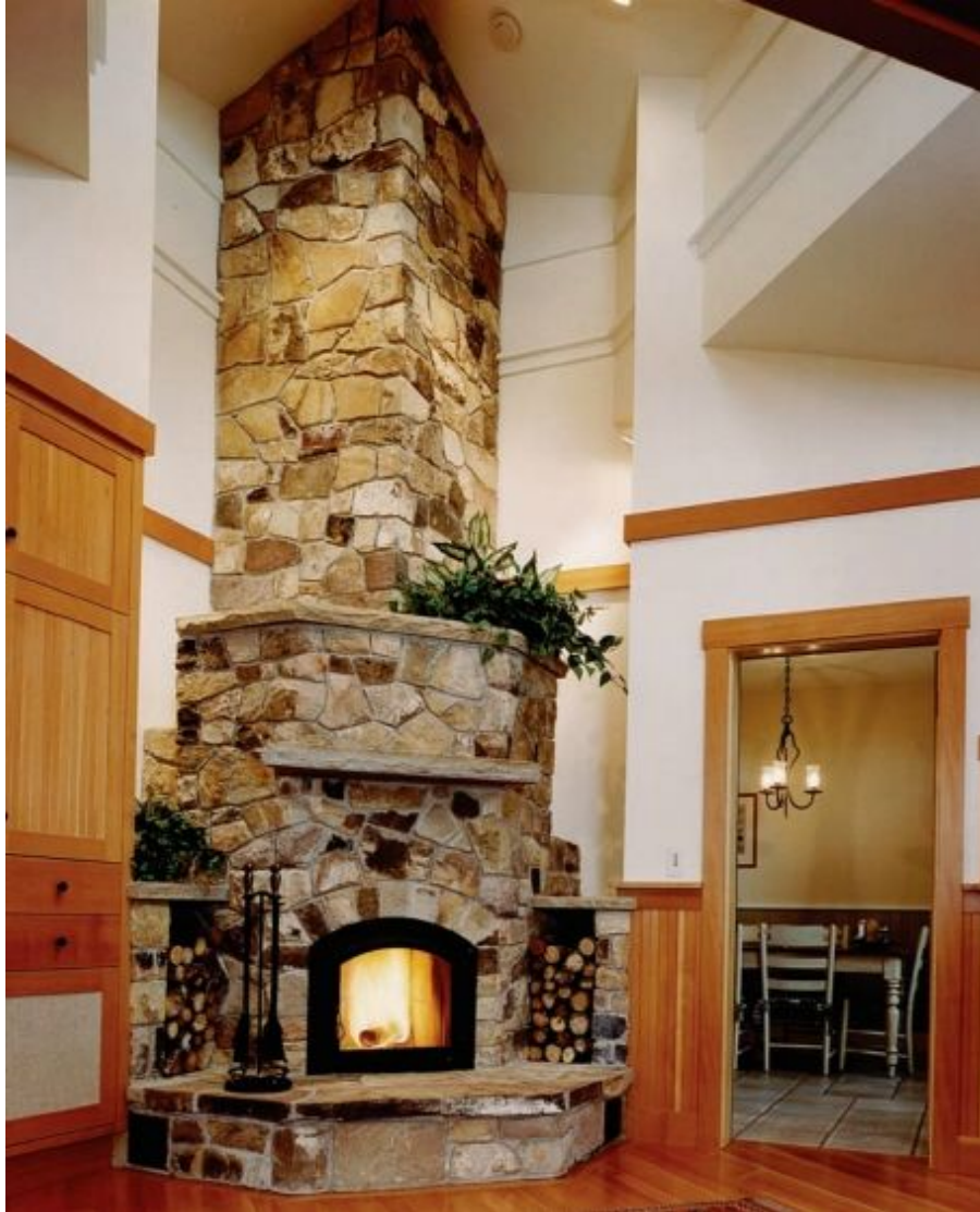
FIGURE 12.1. A massive five-sided stone masonry heater occupies the corner of this central space. The giant chimney hugs the corner all the way to the tall cathedral ceiling. Photo courtesy of Temp-Cast Enviroheat.
