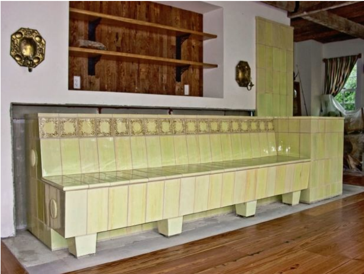
FIGURE 6.18. This entire masonry heater is a sitting area made with structural tiles or kacheln . The firebox is in the far right of the photo, the box-like short structure facing another part of the room. Photo courtesy of New England Hearth and Soapstone.
