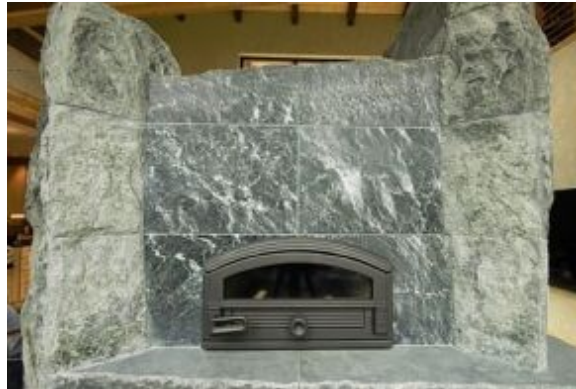
FIGURE 11.11. The shape of the door is often a hint as to the general size of the oven option in a masonry heater. This is the backside of the Tulikivi “boulder” heater shown in figure 9.1. The door is roughly 16 inches wide by 10 inches tall. The oven is only a little larger than this. Photo courtesy of WarmStone Fireplaces and Designs.
