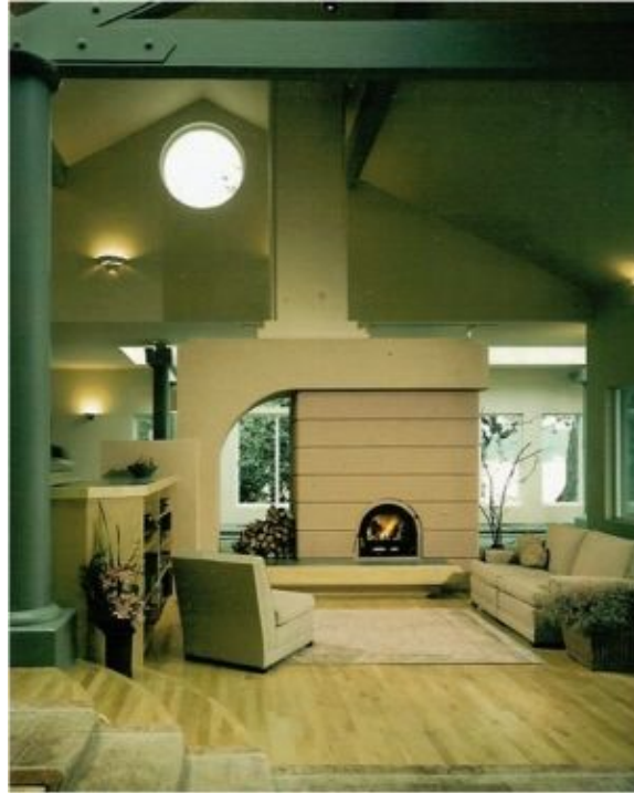
FIGURE 6.9. This chimney attaches to the masonry heater at its top. The chimney for the heater is partially supported by the unheated “leg” to the left of the heater. The stucco has horizontal inset lines to break up the large, flat surface. This photo reinforces that stucco, like tile, offers unending color choices. Photo courtesy of Envirotech Masonry Heaters.
