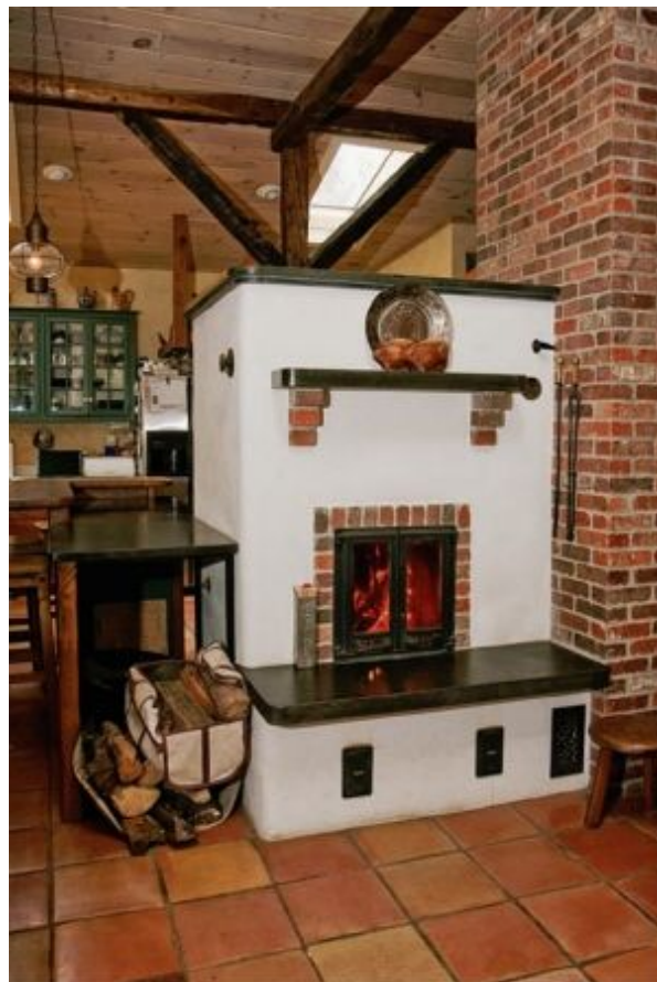
FIGURE 4.3. Brick, stucco, and soapstone combine here to create a pleasing rustic look. The soapstone has been oiled, making it almost black. The heater is well placed, radiating into the kitchen behind and to the left as well as into the living room from where the fire is seen. Photo courtesy of New England Hearth and Soapstone.
