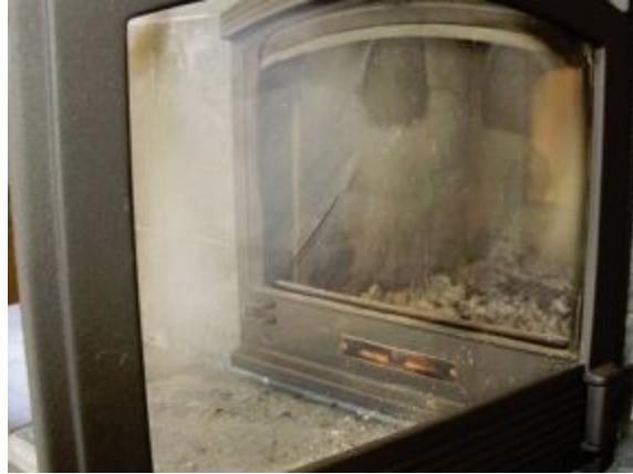
FIGURE 12.6. The fine ash and small amount of soot accumulated on this door over a two-week period. An air wash keeps it mostly clean. The glass can be easily cleaned with a wet cloth dipped in ash.
