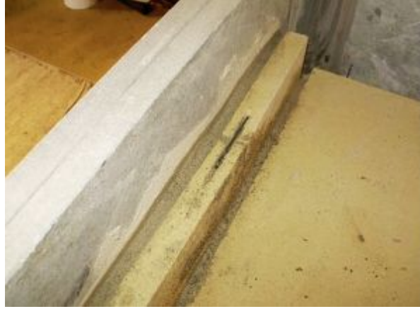
FIGURE 8.38. The entire inner life, whenever possible, is built directly against the exterior “container” of soapstone, assuring ideal heat transfer.
