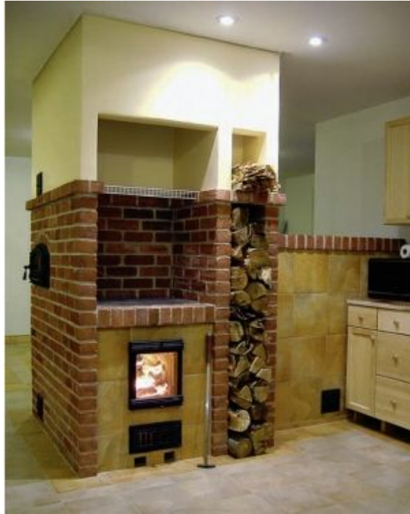
FIGURE 3.9. A unique brick and tile-faced heater built according to the system of free gas movement (see chapter 8 ). The heater incorporates storage and/or work space above the firebox as well as a built-in wood-storage area. On the left side is the door for the integral baking oven. See the other side of this beautiful heater in figure 3.10. Heater designed and built by Stovemaster; photo courtesy of Alex Chernov.
