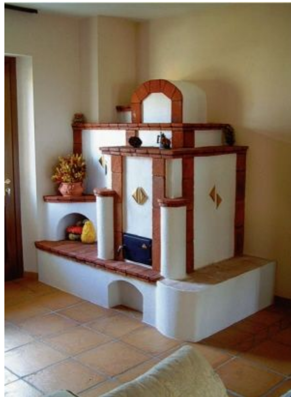
FIGURE 5.6. Like many masonry heaters, this one appears to have no chimney because the chimney is built into the wall. It uses terra-cotta tiles to contrast with stucco, as well as niches and decorative shapes for great appeal. Notice that the black loading door does not have glass. Since a masonry heater is used only for part of the year in most locations, many folks don't want
