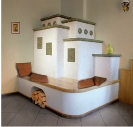
FIGURE 6.16. As suggested in figure 6.15, this masonry heater is a combination of “boxes” containing all the flues in an asymmetric design. Add stucco, tile, some wood for a bench, and a niche for wood storage and you have a beautiful masonry heater. Photo courtesy of Biofire, Inc.
