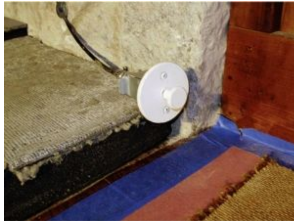
FIGURE 8.11. A close-up of the air-intake control handle, which will be carefully set into the soapstone veneer. The knob pulls out about 1 inch to open.
