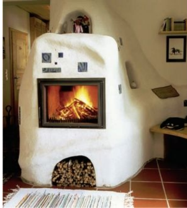
FIGURE 4.18. One distinct advantage of stucco is the ability to make virtually any shape look good. Here an organic, rounded shape is decorated with just a few tiles and purposely imperfectly round arched niches. Notice a sitting area built off the right side of the heater. Photo courtesy of Biofire, Inc.
