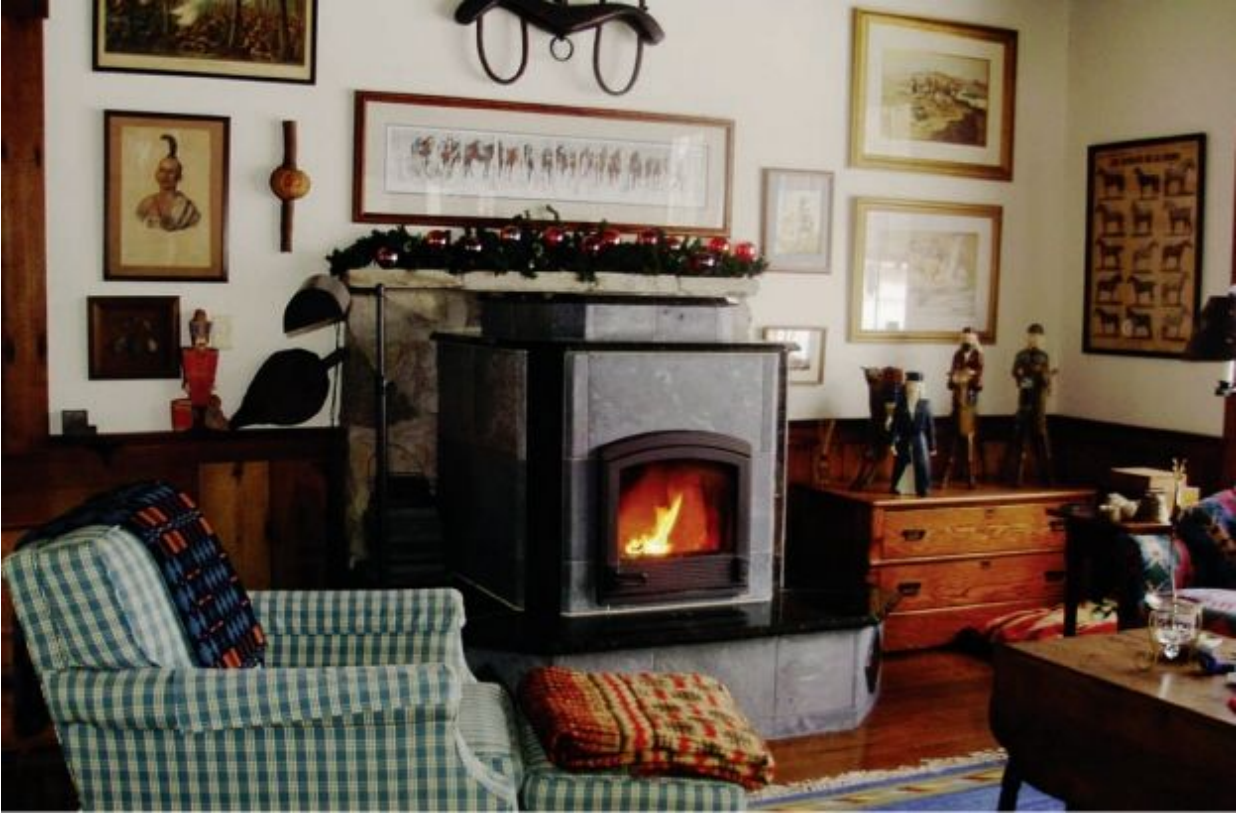
FIGURE 8.53. The heater in its final setting. When this photo was taken, the heater had been in regular use for slightly more than a week. Just prior to lighting a small fire for photos, the heater was checked for temperature. The bench sides, bench tops, and vertical sides of the main body of the heater were uniformly about 135°F; the left rear (where the exhaust first exits the firebox) was higher by about 25°. All the top horizontal pieces, both soapstone and granite, were uniformly at about 110°. These measurements were taken about three hours after the morning fire, which consumed just 28 pounds of fuel.
