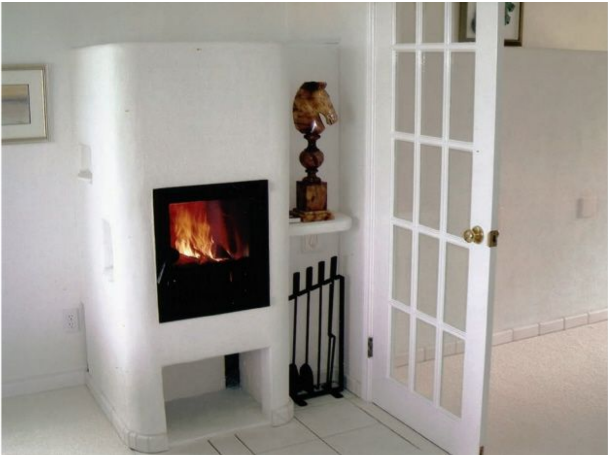
FIGURE 4.12. Here's an example of a way to get the gentle radiant heat of a masonry heater into two rooms separated by doors. The firebox of the heater is in one room, but the bulk of the flues and radiating mass is in the next. Notice small niches in the left side of the stucco heater as well as a generous wood-storage area below the firebox. White tiles form a baseboard. A kachelofen designed, built, and photographed by Ernst Kiesling, Canadian Kachelofen.
