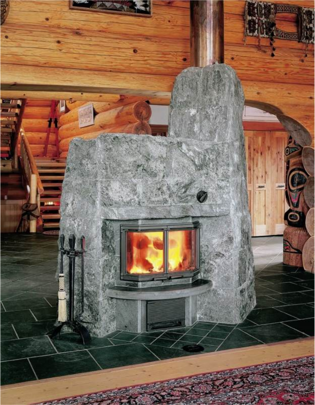
FIGURE 3.7. This massive soapstone heater is meant to resemble a large boulder. The whole veneer consists of large split-faced stones carefully shaped to blend together as if it were one
