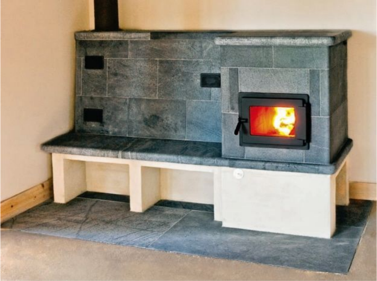
FIGURE 4.11. A relatively small soapstone masonry heater serving double duty as furniture. The entire backrest is heated. The black soot doors reveal that the backrest interior consists of three horizontal flues one atop the other leading to the chimney at upper left. Niches under the seats and firebox could be for firewood, shoes, or other storage. Photo courtesy of New England Hearth and Soapstone.
