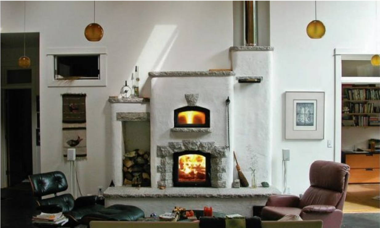
FIGURE 5.7. By properly locating a chimney, you can make sure the smoke always goes up and a white stuccoed heater always stays white. This granite-trimmed heater has an upper-chamber “black” bakeoven. Through the arched bakeoven door glass, you can see the fountain of flame that has just come through the throat from the main firebox below. Notice wood storage to the left and the masonry chimney transitioning to stainless steel on the right. Photo courtesy of Maine Wood Heat Company.
