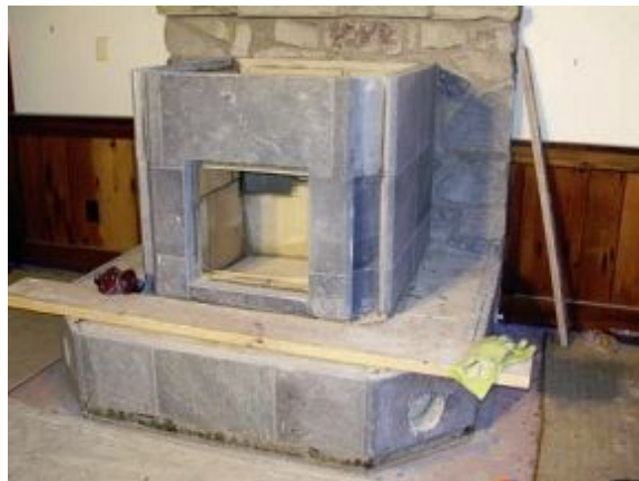
FIGURE 8.43. The container has been lined with more refractory plates pinned together and clay mortared directly to the soapstone. Visible pencil markings indicate centers of flue and locations of remaining linings.
