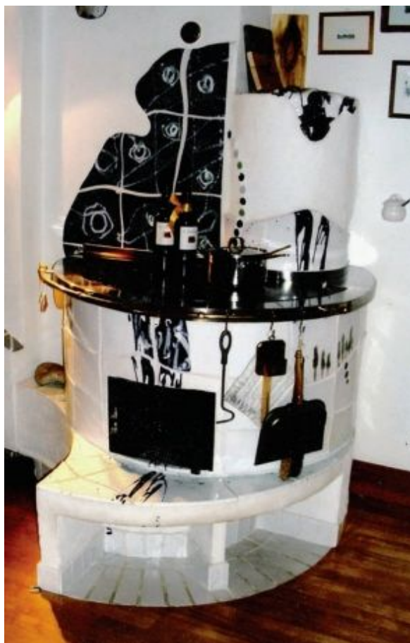
FIGURE 11.20. A unique and functional cookstove and heater in handmade tiles. It isn't often that we see a round cookstove. Kachelofen designed, built, and photographed by Ernst Kiesling, Canadian Kachelofen.
