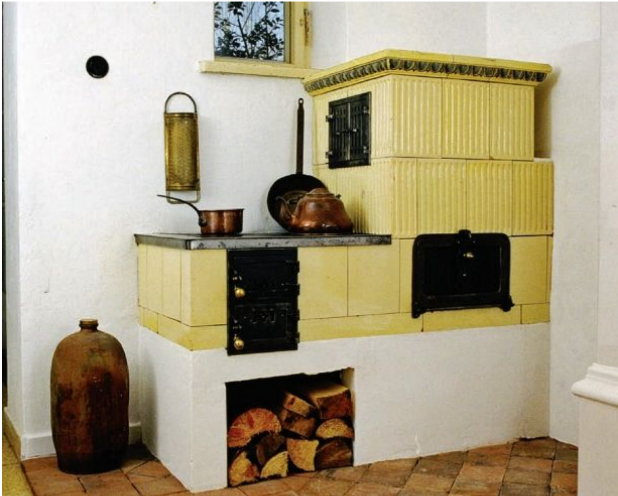
FIGURE 11.10. This is a masonry heater and bakeoven and cookstove—from nineteenth-century Germany! Photo courtesy of Vintage Elements, Greenwood, South Carolina.
