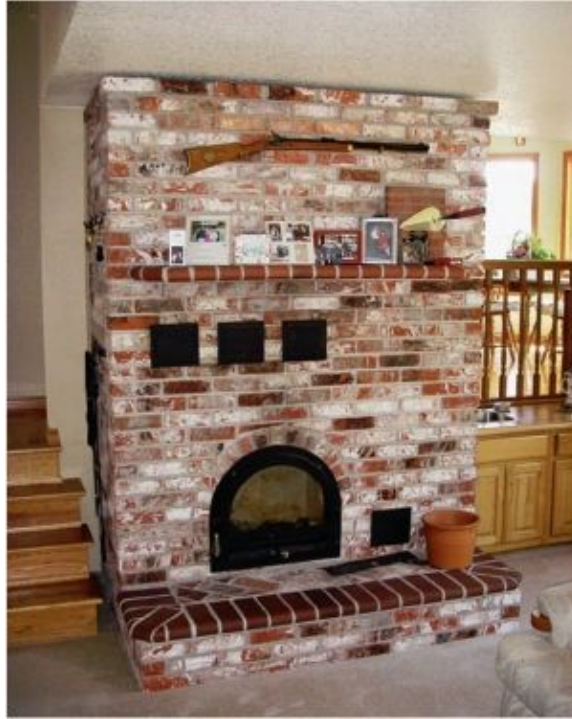
FIGURE 6.11. The firebox is integral with the mass of this heater built using the core kit sold by Envirotech Radiant Fireplaces. Photo courtesy of Envirotech Masonry Heaters.
