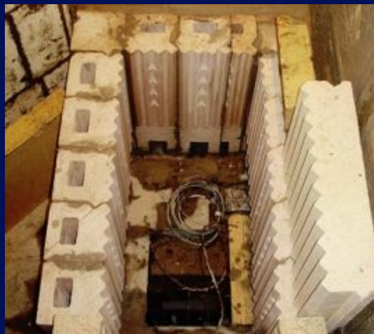
FIGURE 11.6. A good example of a firebox with provision for air supplied to the fire at all levels. What look like columns of the letter A are holes every couple of inches up the height of the firebox walls. Also, the corrugated nature of the wall means that fuel falling against it will not restrict the air supply. Project by New England Hearth and Soapstone.
