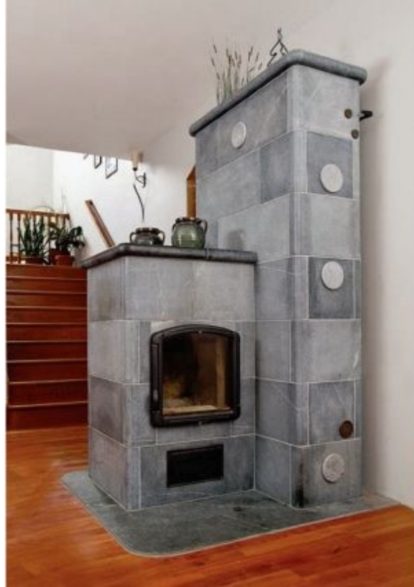
FIGURE 3.2. A unique source of thermal comfort: A vertical heater for vertical people. This custom soapstone heater consists of two primary elements. The firebox is contained in the shorter part; the taller part contains most of the flues. The round “disks” are ash cleanout covers, revealing clues as to where various flues are located. Every flue needs a way to be accessed for eventual cleaning. Photo courtesy of New England Hearth and Soapstone.
