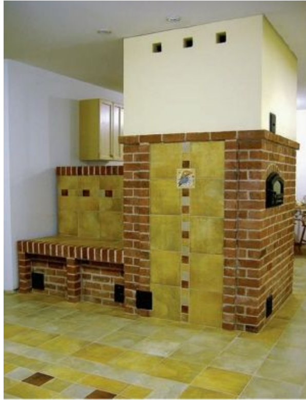
FIGURE 3.10. This is the backside of the heater shown in figure 3.9. The bakeoven door is on the right, and heated seating on the far left. Notice how the tile pattern is echoed in the floor. It's a lifetime, heirloom heater. Heater designed and built by Stovemaster; photo courtesy of Alex Chernov.
