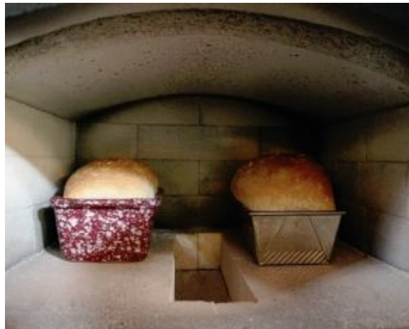
FIGURE 11.13. Between the baking loaves of bread is the throat of this Finnish masonry heater. Project by Maren Cooke and Ken Matesz; photo by Maren Cooke.
