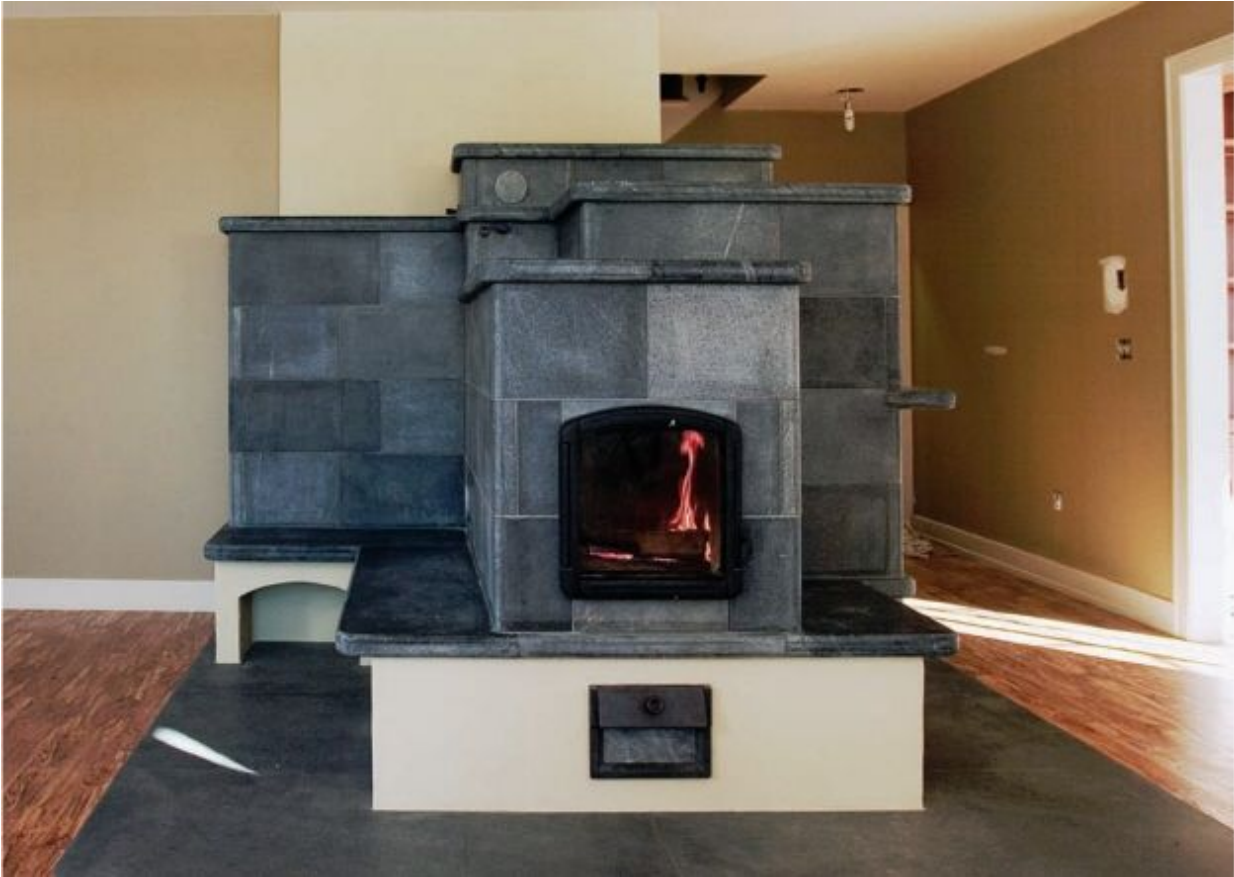
FIGURE 4.16. A very large soapstone-and-stucco heater complex. Notice the multiple levels and asymmetry. To the far right can be seen, at middle, a shelf that sits under a bakeoven door. As with many masonry heaters, the chimney is not visible at all. There is another view of this heater in figure 6.39. Photo courtesy of New England Hearth and Soapstone.
