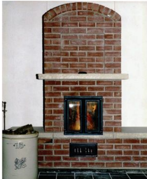
FIGURE 5.2. This masonry heater was built in a basement because it was remodeled and became a primary living space. The red-brick heater features a limestone mantel as well as limestone-capped heated wing benches on either side. The bricks in the center square above the mantel are slightly inset. The owner plans to one day put handmade tiles here.
