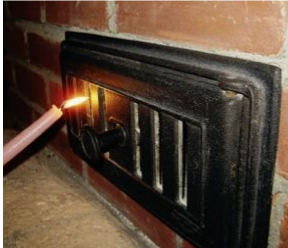
FIGURE 11.3. Notice how the flame of the candle is pulled horizontally into the heater—a sure sign of good positive draft. It's wise to do this test before lighting a large load of wood.
