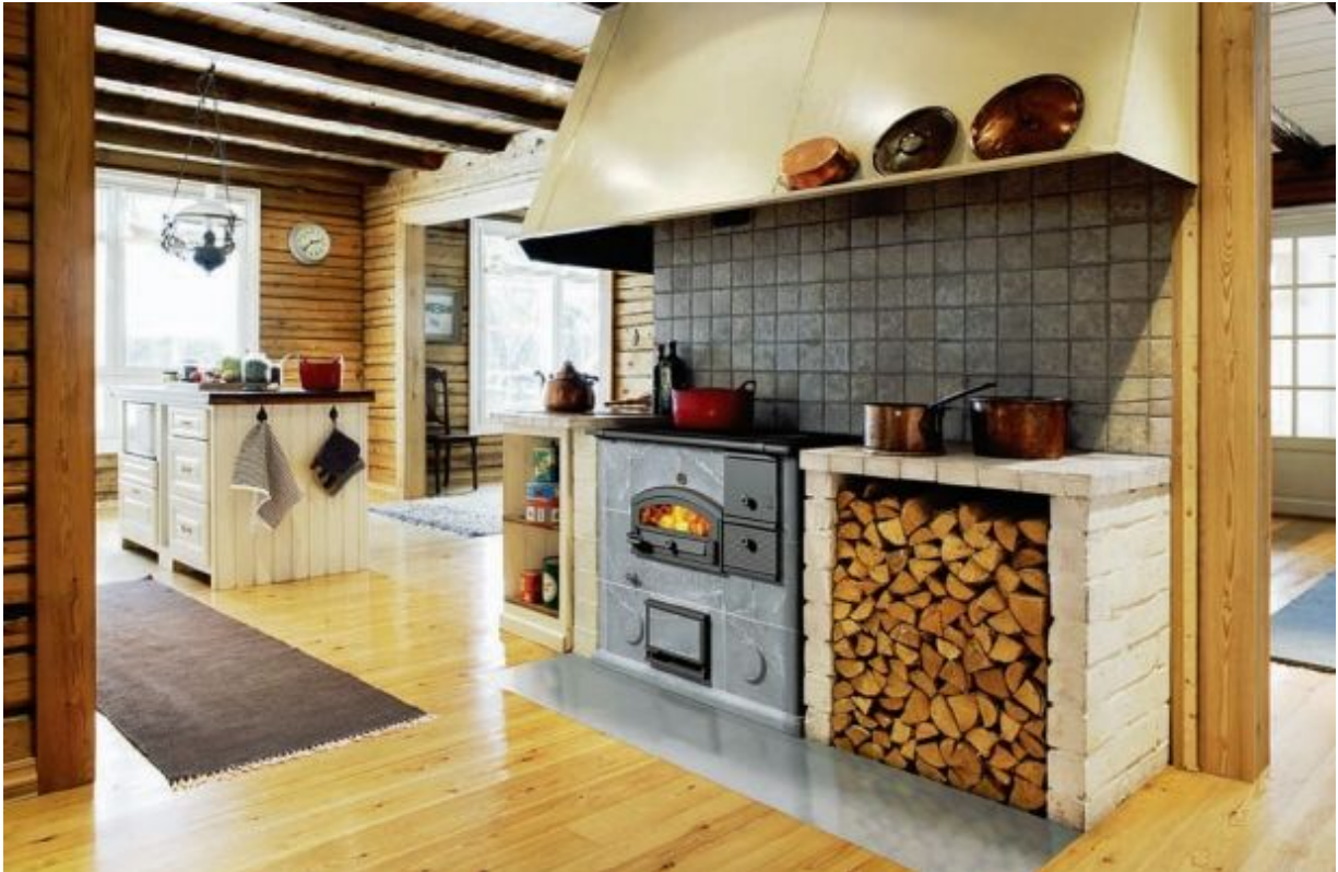
FIGURE 11.18. A well-designed masonry cookstove adds tremendous versatility to heating with wood. This model has both a functional cooktop and a bakeoven that can be fired separately. Photo courtesy of Tulikivi Corporation.
