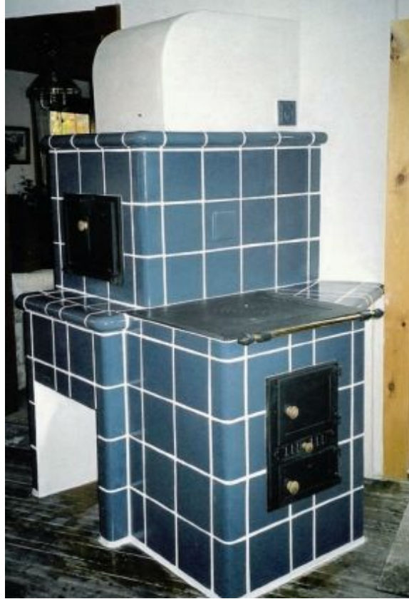
FIGURE 11.21. An all-tile heater, oven, and cookstove designed, built, and photographed by Ernst Kiesling, Canadian Kachelofen.
