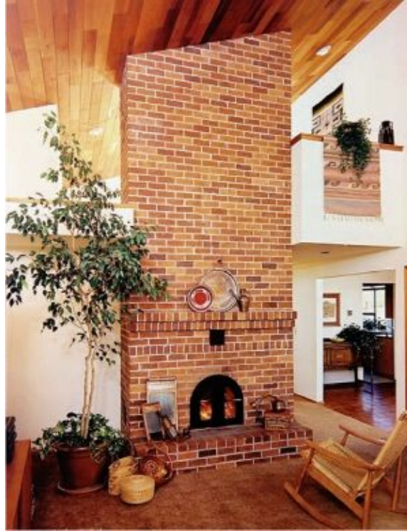
FIGURE 6.30. Common brick is an oft-used material for masonry heaters. Photo courtesy of Envirotech Masonry Heaters.
