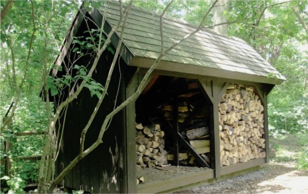
FIGURE 10.10. A well-built, roofed wood shelter. This shelter has solid sides on all but one side, other shelters use latticework so more wood is exposed to the drying effects of the wind.
