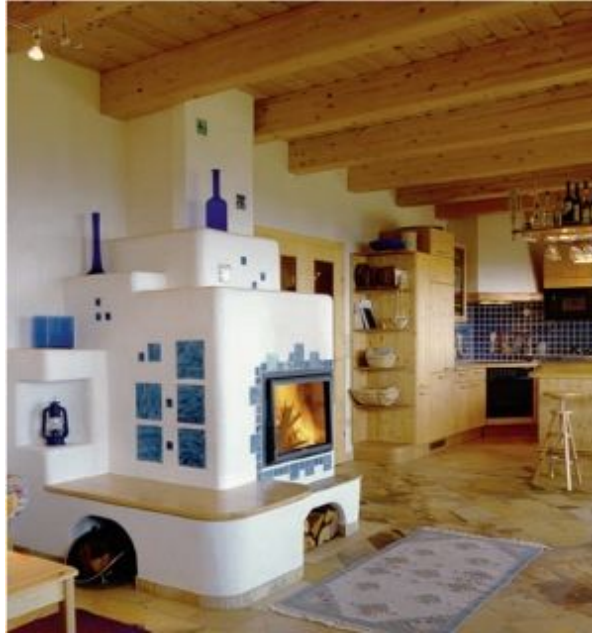
FIGURE 3.13. A masonry heater warms every thing that it “sees.” This one sees both the living and dining areas from its central location. The asymmetric shape provides varying levels for placing decorative objects. Tile accents complete the unique look. Under the wood-topped benches are niches for storage of wood or other items. Notice how the chimney becomes part of the asymmetry and decoration. Photo courtesy of Biofire, Inc.
