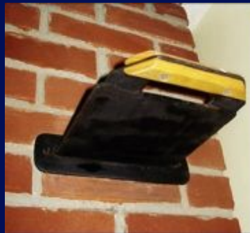
FIGURE 7.12. An example of a guillotine damper pulled out to open the flue.
