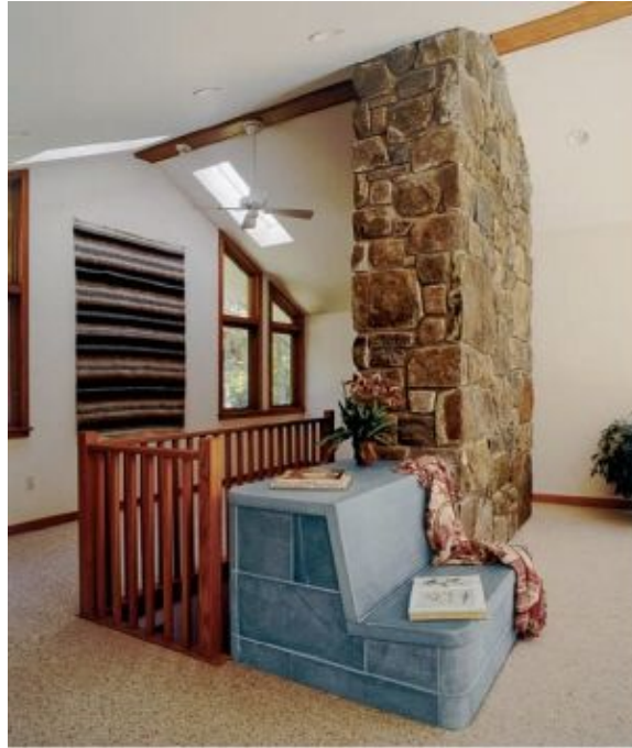
FIGURE 6.23. This soapstone heater extends through the ceiling into the second floor. It's one version of a two-story heater. | FIGURE 6.24. Here is the second-floor portion of the heater shown in figure 6.23. Having the heater extend into another level of the house provides radiant heat to that upper level. In this case it's a simple seat, though it could have been designed to be larger or taller with more heating capacity. Photo courtesy of New England Hearth and Soapstone.
