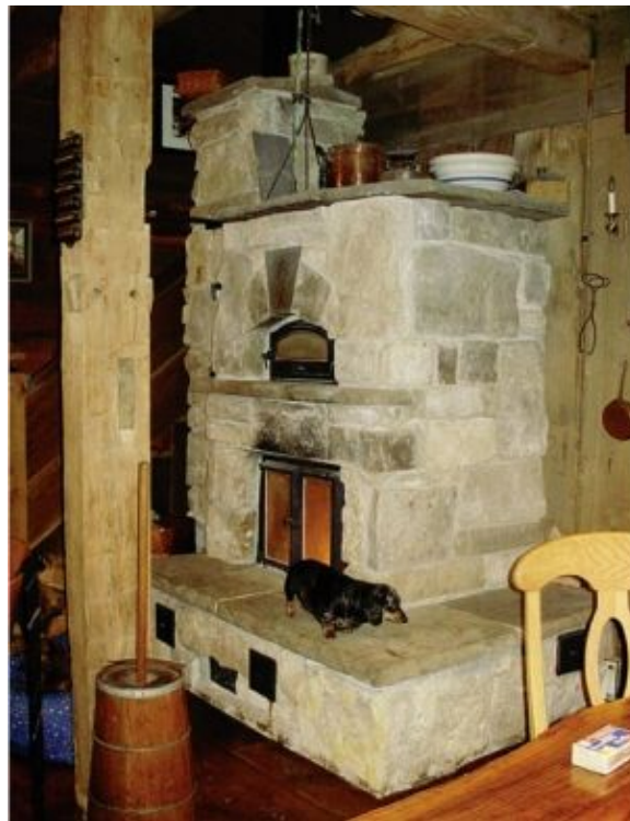
FIGURE 6.35. An owner-veneered limestone masonry heater. The sandstone slabs used over the heated benches and as the capping stones at the top of the heater are from an old sidewalk.
