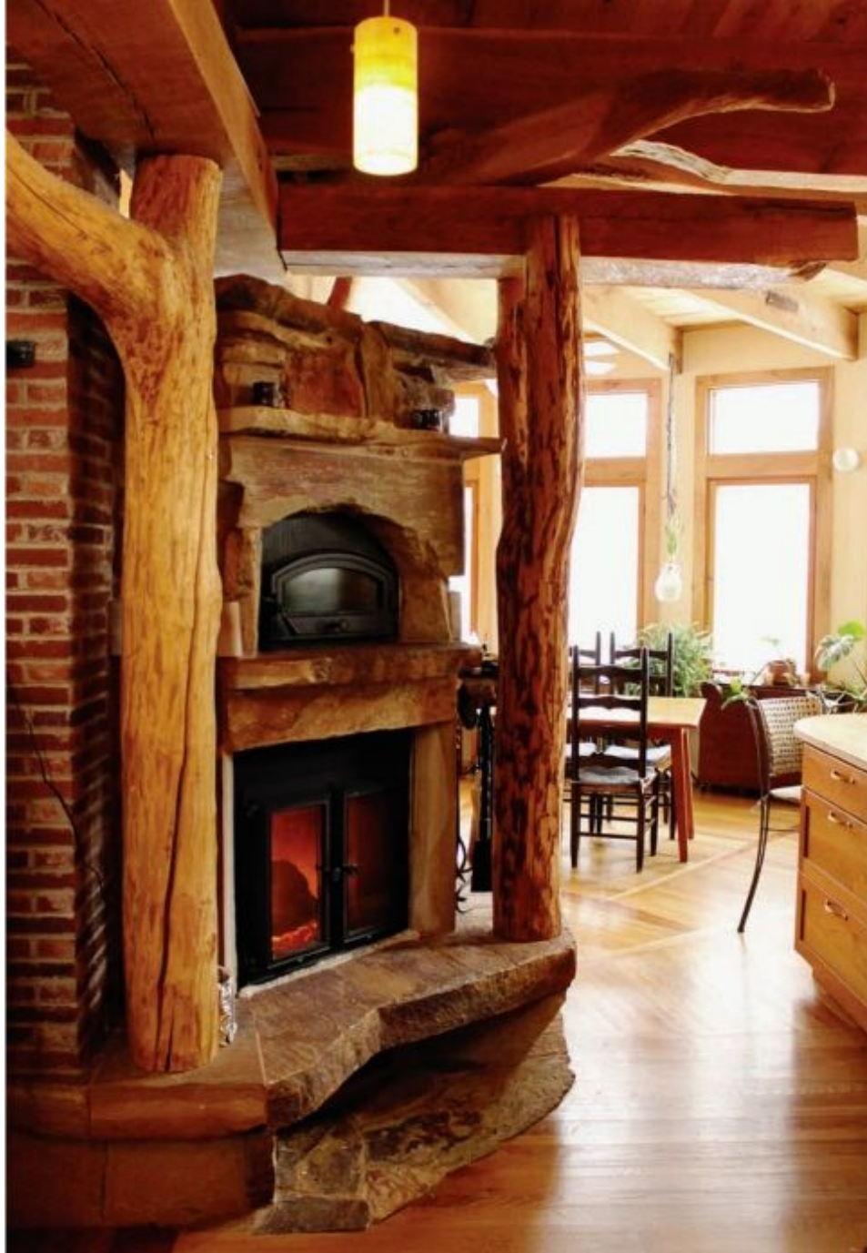
FIGURE 3.1. This unusual red sandstone masonry heater was designed on the fly, piece by piece. It incorporates 5-inch-thick sandstone slabs for the raised hearth—all cut from the same huge slab of stone. Some of the “scrap” from that (some scraps measured 2 or 3 feet square) formed the upper veneer of the heater below the level of the bakeoven. Other views of this heater can be seen in figures 6.31, 6.36, and 6.43. Heater by Maren Cooke and Ken Matesz; photo by Maren Cooke.
