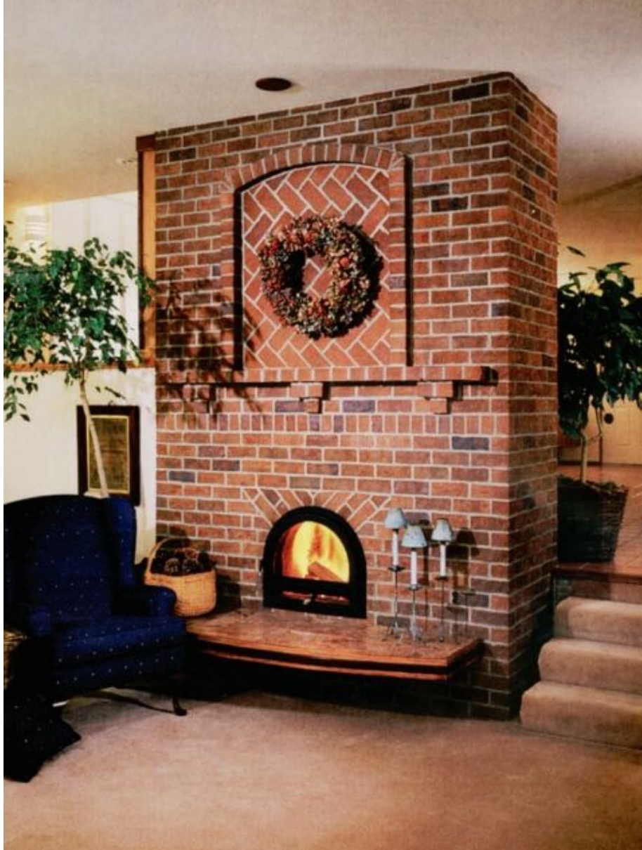
FIGURE 7.1. This is a very straightforward, elegant, and well-placed brick masonry heater. Notice the inset herringbone brick pattern above the mantel. The heater was built all the way to the ceiling, giving the impression of the huge mass continuing on, though the workings of this heater end about 1 foot below the ceiling. Photo courtesy of Envirotech Masonry Heaters.
