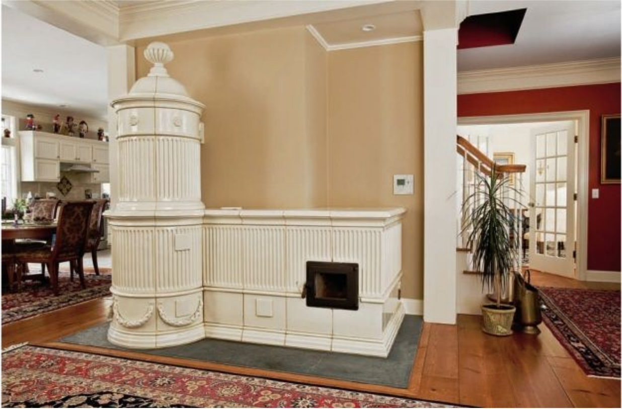
FIGURE 2.1. A modern-day kachelofen with traditional elements graces this Connecticut home. The fluted tiles and cylindrical element with braids and rosettes hark back to another century. Yet this heater boasts a computer-controlled combustion air supply and an efficient internal design facilitated by both a craftsman's experience and computer modeling. Photo courtesy of New England Hearth and Soapstone.
