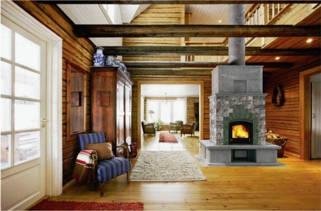
FIGURE 7.11. This massive soapstone masonry heater has split-rock-faced stone accents and a green serpentine arch. Notice the shallow niche above the wraparound mantel and cylindrical stone wrapping the chimney flue. The heater is perfectly placed in the middle of the primary living space. Photo courtesy of Tulikivi Corporation.
