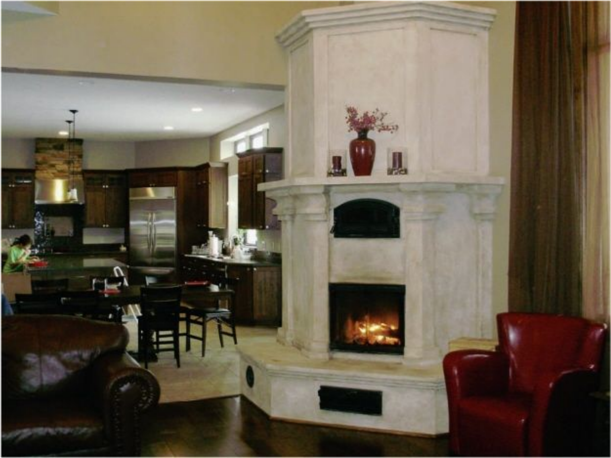
This masonry heater has an oven (the upper, arched door). The heater is finished in finely detailed stucco. The customer wanted a relatively conventional fireplace look blended with a five-sided corner-heater design. Three sides are visible here while the two back sides fit squarely in the corner.
