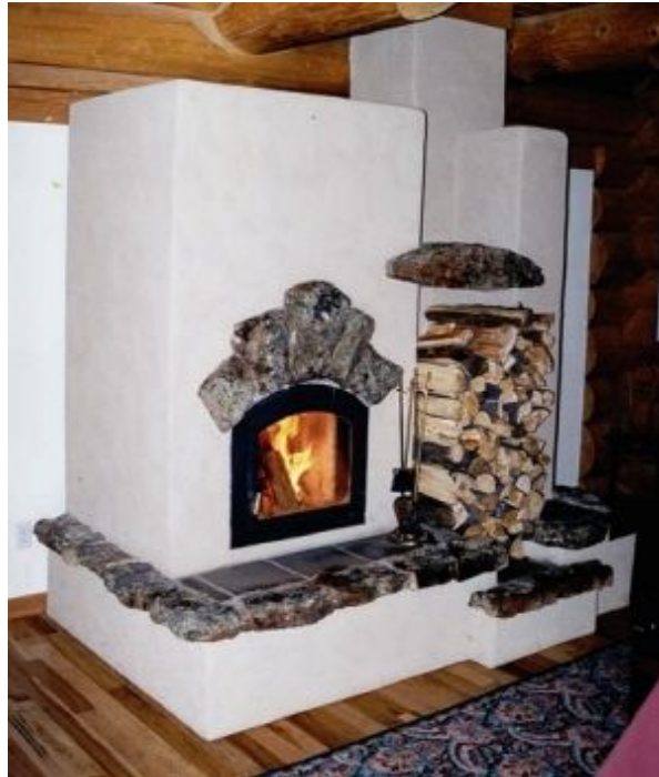
FIGURE 1.3. Stucco and stone combine in this large heater. Notice how the chimney is separated from the heater itself by a wood-storage area. The heater and chimney are tied together above the wood-storage alcove with a long curved stone. Fire, stone, and wood are basic natural elements and have a strong effect on human beings—sometimes at an unconscious level. Photo courtesy of Temp-Cast Enviroheat.
