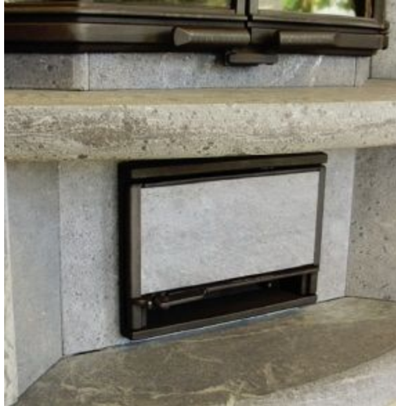
FIGURE 12.2. If equipped, the ash box door is usually right below the firebox.
