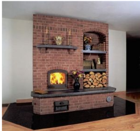
FIGURE 3.8. This unique brick-and-soapstone heater features a spacious raised hearth. The bench surface, mantel, and shelves are all made of soapstone. The built-in wood storage and shelves provide both visual interest and practical storage. An arched door and matching arch over the niches are an elegant touch. Photo courtesy of New England Hearth and Soapstone.
