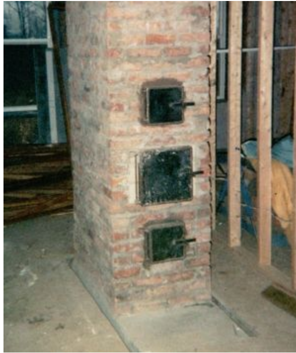
FIGURE 2.13. A brick, single-skin (meaning the inner life and veneer are one-and-the-same, see chapter 8 ) heater built using Basilio Lepuschenko's plans. The doors, from bottom up, are ash cleanout, fuel-loading door, and soot door. The heater was subsequently stuccoed white. Photo by Dean Witt.
