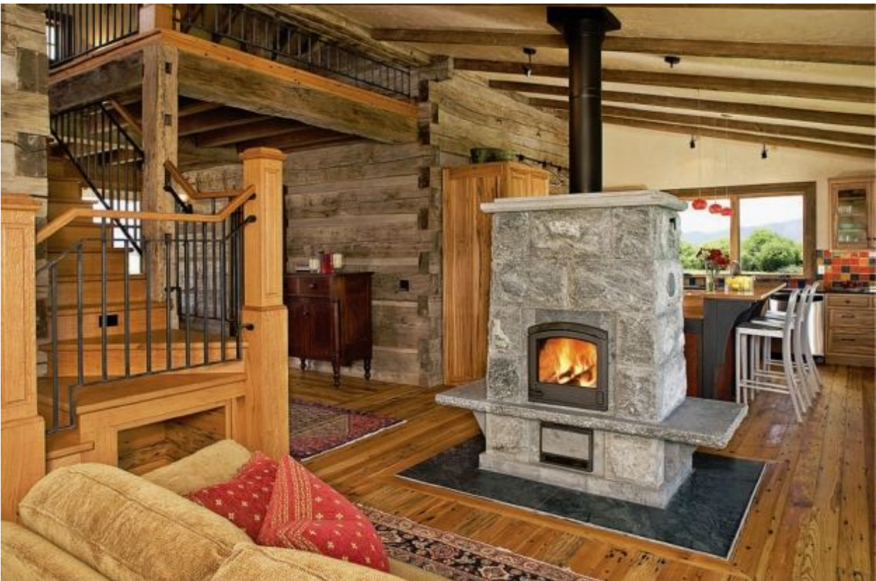
FIGURE 5.5. Here is an heirloom-quality soapstone heater perfectly located for enjoyment and heating of the living space. Large split or rock-faced soapstone blocks create a gently tapered
