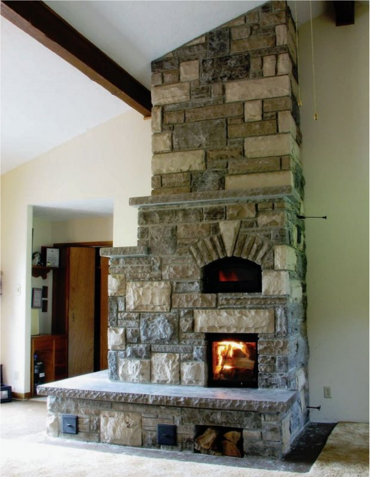
As you can imagine, given the fact that combustion gases will fully occupy a volume of any shape or size, the system of free gas movement
