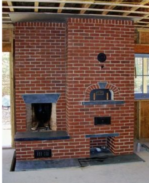
FIGURE 6.29. The bakeoven, inside the low arched door, is strictly for baking and not for heating. Photo courtesy of Maine Wood Heat Company.
