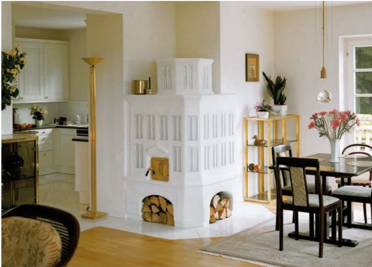
FIGURE 6.33. A highly refined look achieved with stucco, a versatile material. It’s used in a simple, compact design with clipped corners and a small “cupola” on top. Note the small loading door on the left and the abundant wood storage. Photo courtesy of Biofire, Inc.
