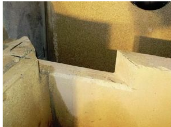
FIGURE 8.29. The start of the “outburn” from the firebox, which is the exit from the firebox into the first vertical flue. The skew cuts direct the exhaust of the fire to the flue that is snugly built into the back left corner of the heater.
