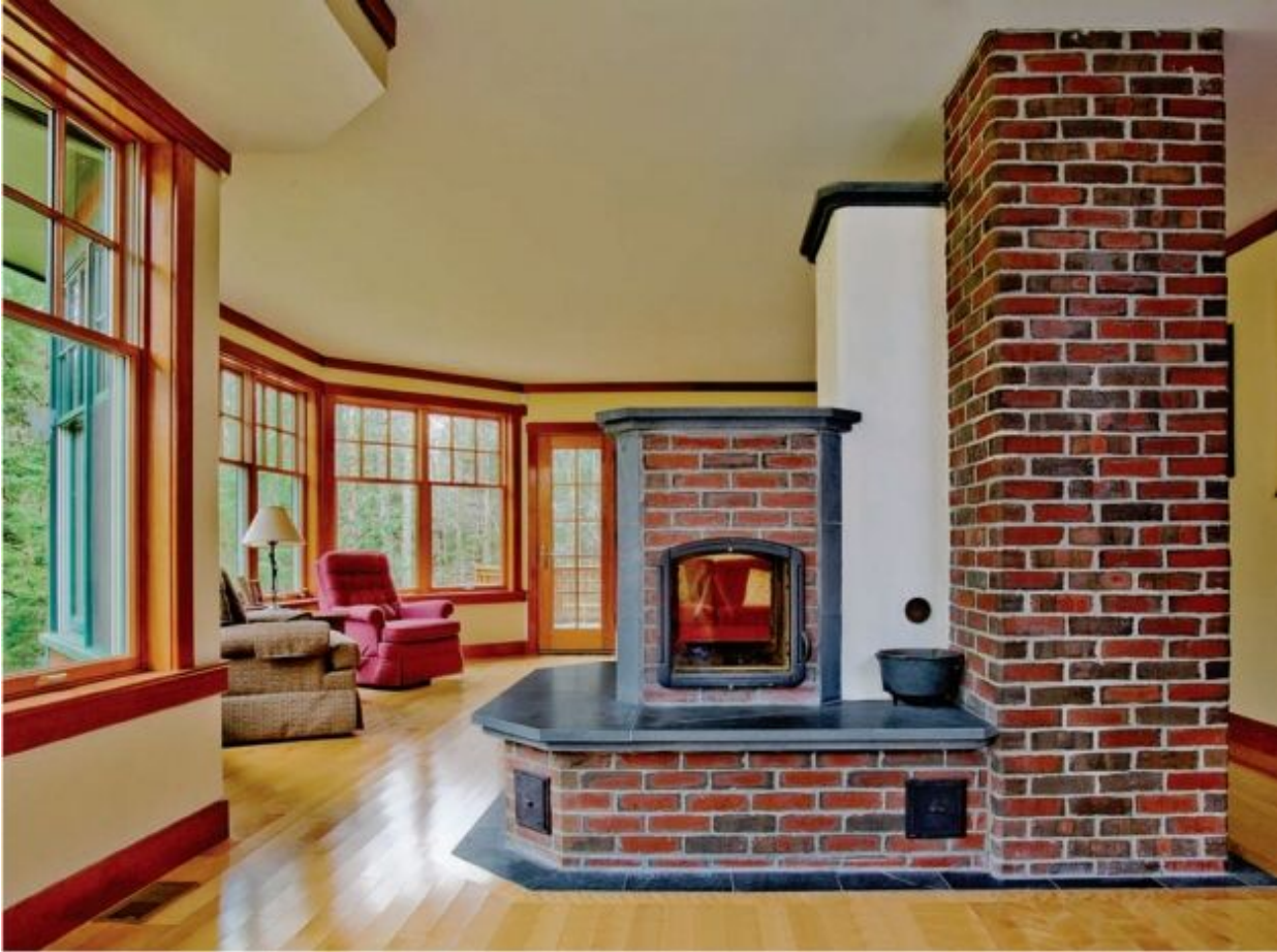
FIGURE 1. Who wouldn't want the sun shining in their home every day? This brick, stucco, and soapstone heater gently separates a living room from a dining room. The brick chimney is in the right foreground; the soapstone-topped benches contain flues that make these warm seats. The stucco mass behind the chimney contains more flues for heat storage. Photo courtesy of New England Hearth and Soapstone.
