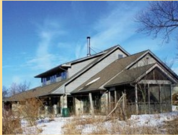
FIGURE 1.11. Although it looks a lot like a typical house, the Tuer/Paskewitz residence is a functional passive solar and earth-bermed home. Photo by Tom Tuer.
