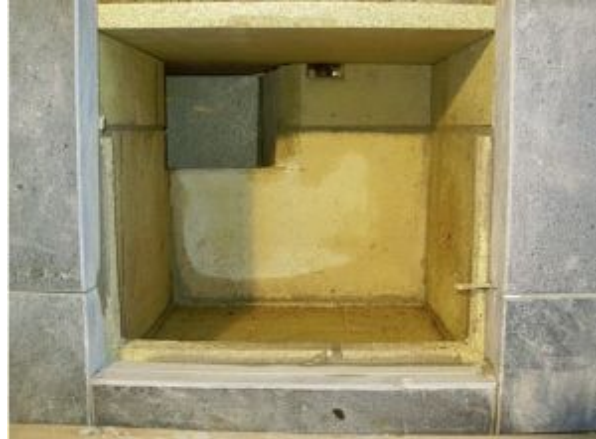
FIGURE 8.36. A view through the firebox door opening. Visible are the insulation board, the gas slot and flue behind, and the outburn to the left. Note how the soapstone at the door opening is fully protected from intensely hot fires by refractory plates that create an opening slightly smaller than the soapstone opening.
