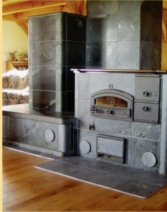
FIGURE 7.18. The cookstove/bakeoven unit in the foreground gets occasional use while the main heater, center left—facing the living room—is the primary heat source for this 2,000 square foot home. Tulikivi by Masonry Heater Store. Photo by Erich Gundlach.
