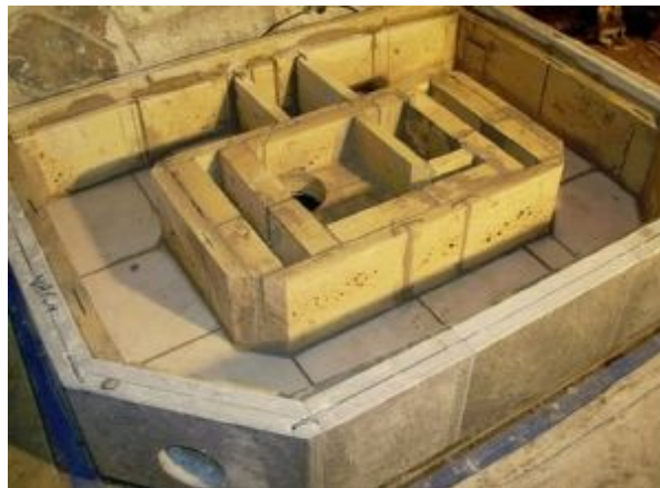
FIGURE 8.22. A perspective view of the base course of the inner life. The two parallel plates behind the support structure mark the beginning of the two vertical flues that are located behind the firebox.
