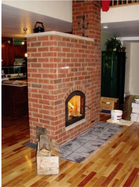
FIGURE 8.59. A Crossfire masonry heater just after completion. Notice how narrow it is. No other standard kit makes a heater this narrow. Photo courtesy of Crossfire Fireplaces.
