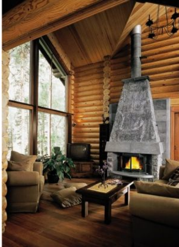
FIGURE 3.14. A heater is a real radiant heat source, like the sun. It actually warms people and the house, not just air. This soapstone heater features split stone and massive smooth stones above the firebox. A multi-sided door enhances fire viewing. Though the upside-down funnel shape gives the impression of smoke going straight from the firebox up the chimney, this is a real masonry heater that redirects the exhaust through flues before it gets to the final exit. Photo courtesy of Tulikivi Corporation.
