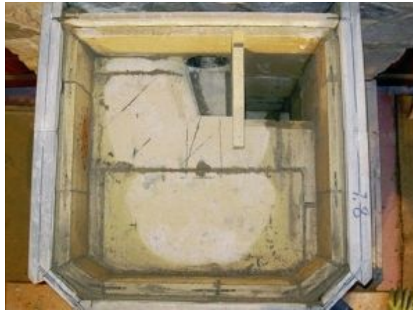
FIGURE 8.43. The container has been lined with more refractory plates pinned together and clay mortared directly to the soapstone. Visible pencil markings indicate centers of flue and locations of remaining linings.
