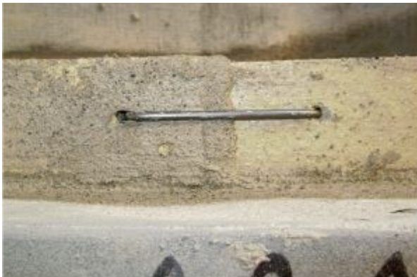
FIGURE 8.16. A view of the same cleanout seen in figure 8.15, this time through the soapstone opening as you would see it after the heater is done (minus the eventual soot door).
