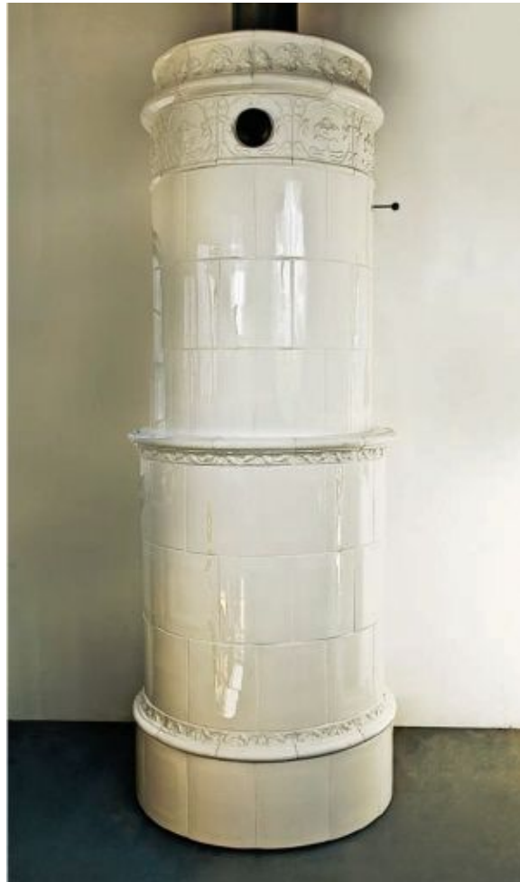
FIGURE 6.5. The tall cylindrical style of a traditional kachelugn . Note the intricate braids and textures cast into the tile, especially at the top. Photo courtesy of New England Hearth and Soapstone.
