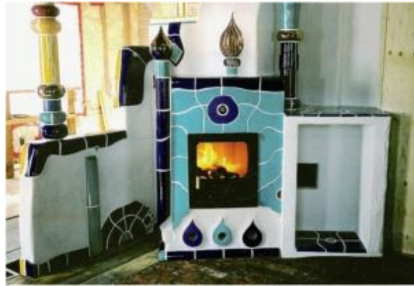
FIGURE 3.6. Front view of the heater shown in figures 4.8 and 8.1. This kachelofen was designed, built, and photographed by Ernst Kiesling, Canadian Kachelofen.
