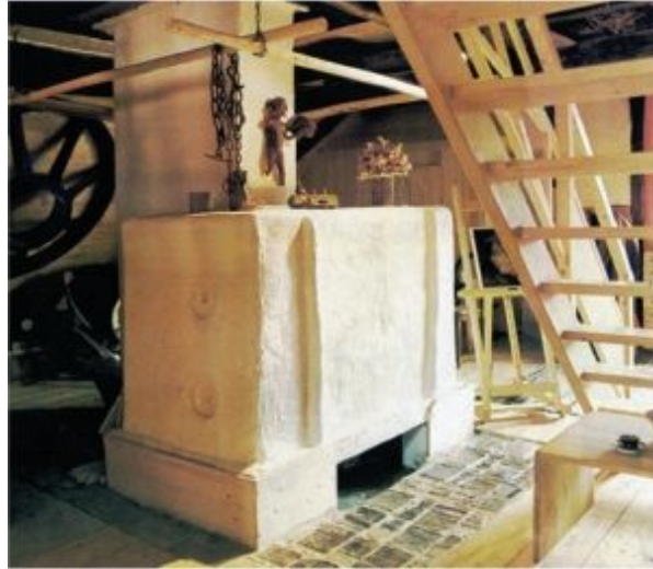
FIGURE 1.8. Here is a simple stucco heater centrally located in the living space. The open stairway allows the radiant heat to reach all areas of the room. Notice the drying racks above the heater and around the chimney mass. Photo courtesy of Biofire, Inc.
