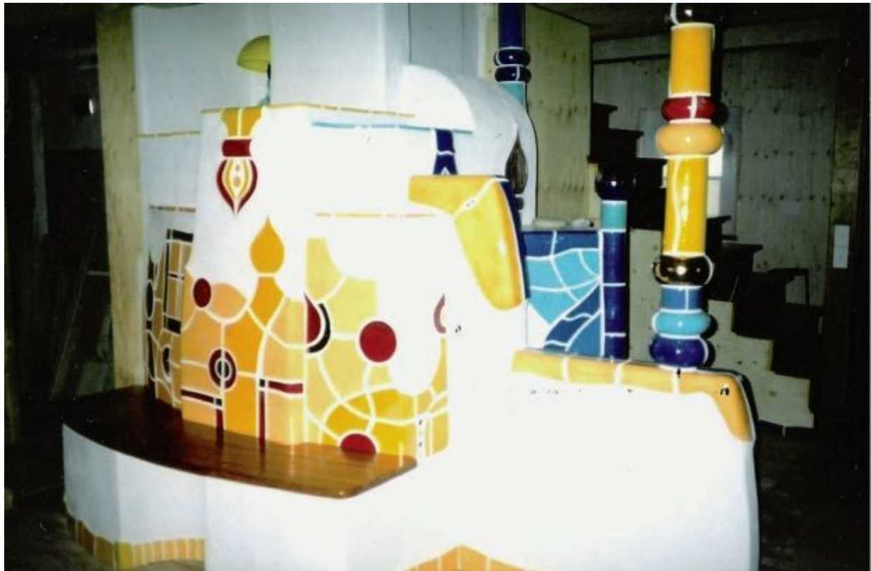
FIGURE 8.1. This is the backside of the heater seen in figures 3.6 and 4.8. The handmade tiles forming the backrest of the wooden seat create a picture of spires similar to the actual ones that exist over the firebox. Combining handmade tiles with handcrafted heaters means an infinite range of possible designs. Kachelofen designed, built, and photographed by Ernst Kiesling, Canadian Kachelofen.
