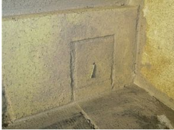
FIGURE 8.15. The inner life is begun with a layer of 11.2-inch refractory plates. The little square is a cleanout access cut into the plate. Behind the square is the circular opening in the soapstone seen in figure 8.16. The square cleanout piece has a shaped wire handle, seen bent against the inside here.
