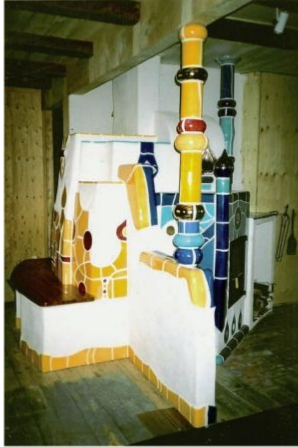
FIGURE 4.8. The firebox of this heater is to the right and the wood-topped sitting area to the left. All the mass between contains the flues and radiates heat. Notice the hand-painted, handmade tiles. This heater is also seen in figures 3.6 and 8.1. This kachelofen was designed, built, and photographed by Ernst Kiesling, Canadian Kachelofen.
