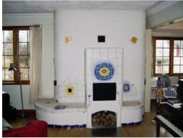
FIGURE 10.3. This tile-and-stucco heater has handmade and hand-painted tiles. Both the seat and the mass behind the tiled firebox are for heat storage. Kachelofen designed, built, and photographed by Ernst Kiesling, Canadian Kachelofen .
