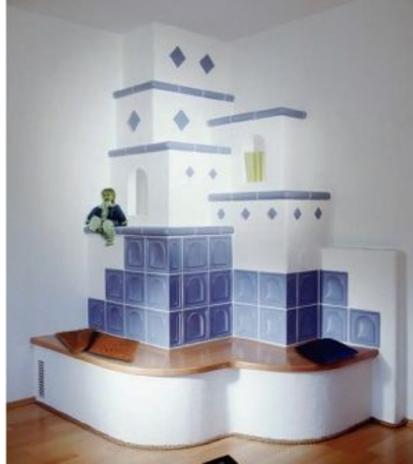
FIGURE 4.5. The corners of rooms are usually occupied by furniture. This masonry heater is warm furniture and art at the same time. By building with multiple tiers and sides, a lot of radiating surface fits in a small area and creates visual interest. Notice the small niches repeating the shape of the glazed tiles. The wooden bench surface is comfortable to sit on even when the heater is not in use, while stone or tile surfaces might feel cold at those times. Photo courtesy of Biofire, Inc.
