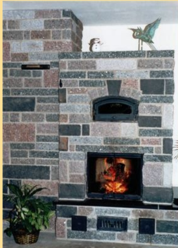
FIGURE 1.12. A granite masonry heater serves as the sunshine when the real sun hides behind clouds at the Tuer/ Paskewitz passive solar residence. Stove by Masonry Heater Store, LLC; stonework by Peter Skove; photo by Nancy Matesz.
