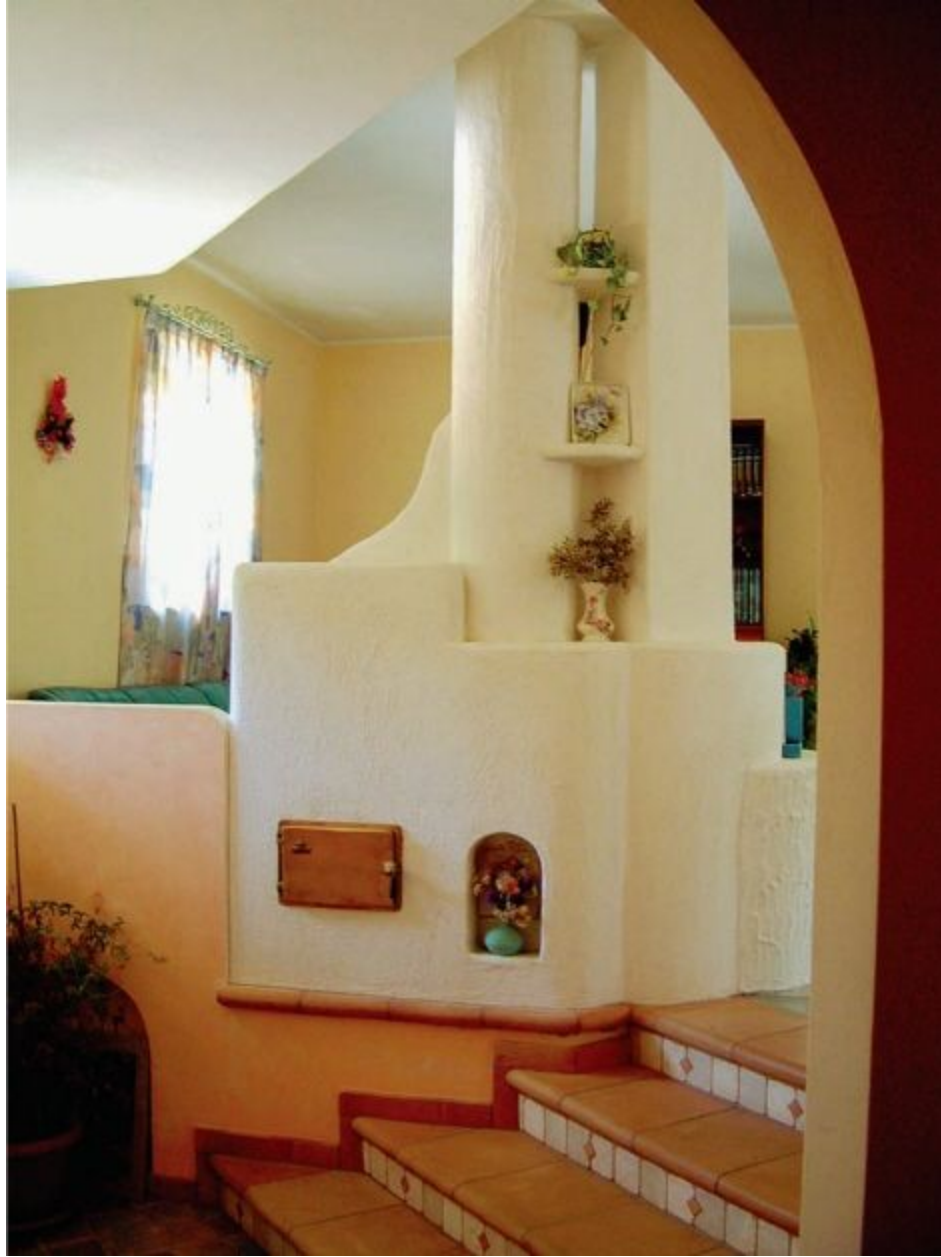
FIGURE 10.1. A stucco heater centrally located in the home. The loading door at lower left is at waist level for easy loading without bending over. Niches, shelves, and curved elements add visual interest and a place to set decorations. Photo courtesy of Biofire, Inc.
