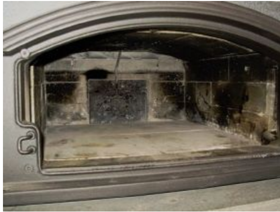
FIGURE 11.15. A white/black hybrid oven can be used either as a combustion chamber or as a white oven. In the center back of the oven is an ash dump door. In the upper back is a damper to open the oven to the flues of the heater when used as a combustion chamber.
