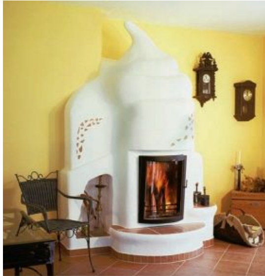
FIGURE 6.6. Free-form shapes can be made with the use of stucco. Delicate splashes of color dot this heater, which almost looks like ice cream in a cone. Niches and continuous changes in size add yet more interest. Photo courtesy of Biofire, Inc.
