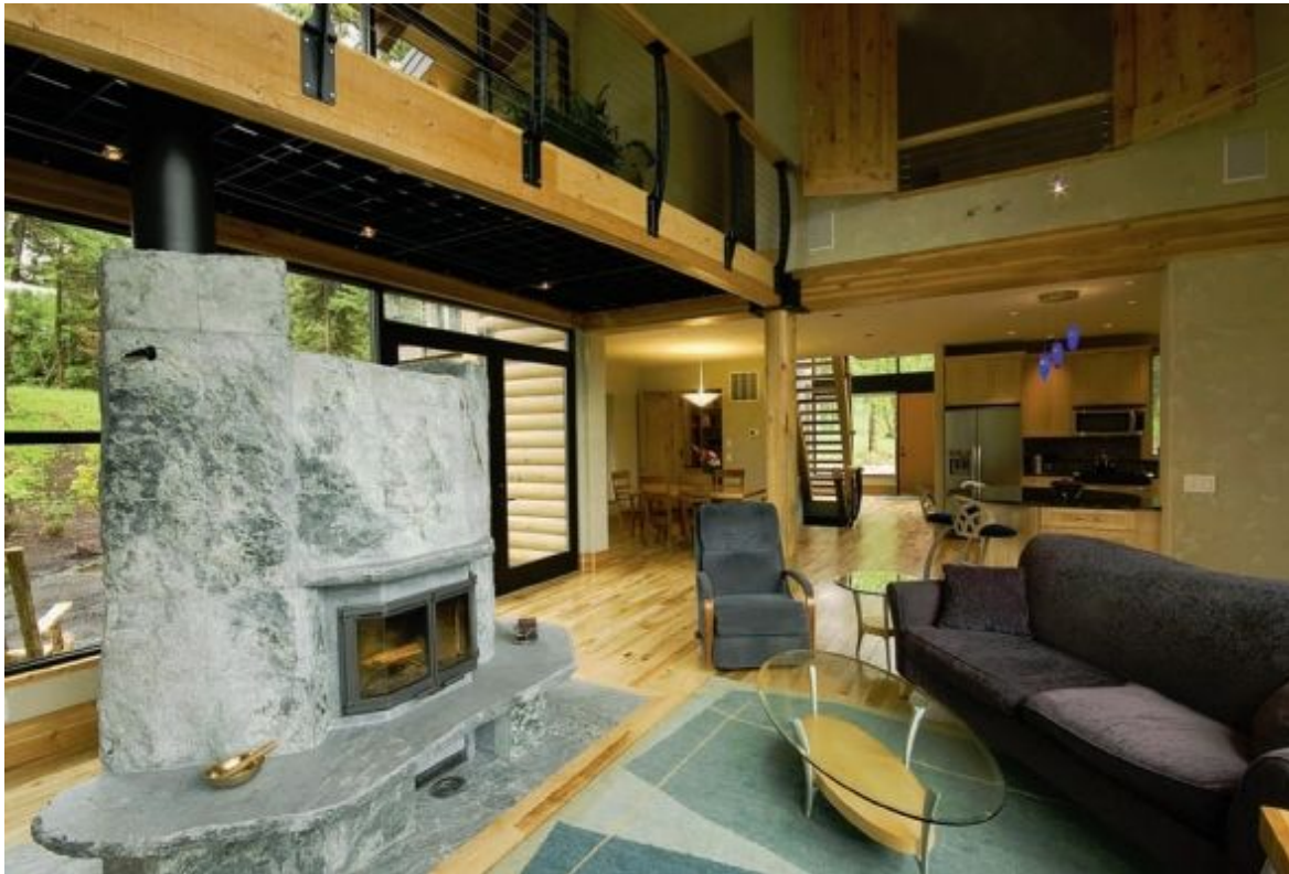
FIGURE 9.1. A Tulikivi boulder heater is the focal point in the center of this home. Note the broad raised hearth with natural, free-form edge. The backside of this heater is shown in figure 11.11. Photo courtesy of WarmStone Fireplaces and Designs.
